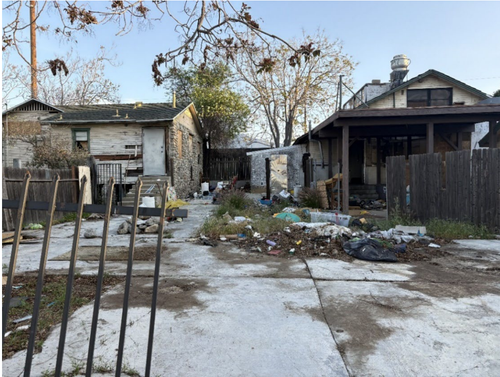
Photo 9: Site overview. View of the abandoned structures and refuse onsite, facing north.
