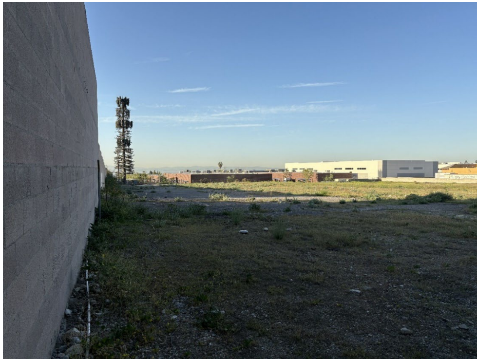
Photo 2: Site overview. View of the site from the northeastern section of the parcel, facing south towards West 11 th Street.
